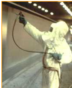
Spraying paint on a steel bridge beam
